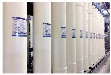
UF/RO system designed and constructed by WesTech Engineering (WWW.WESTECH-INC.COM)
